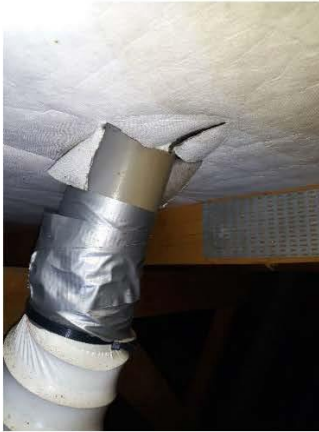
Woven polypropylene roof membrane
